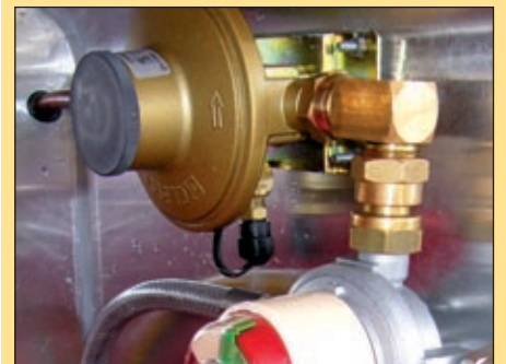
Option 2 Fit an 01-1755 automatic changeover head using a 01-1677 right angled adaptor. Height has been lowered so use Stainless Steel 01-6050SS.
